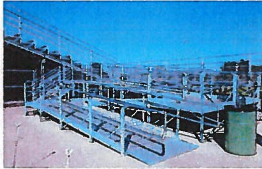
Typical aluminum ramp structure
