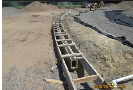
Inner curb and trench drain formwork
