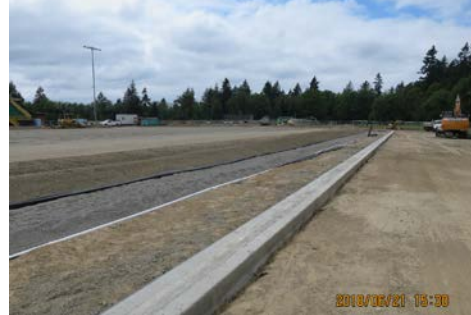
Poured curb and drain
